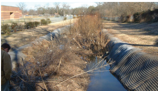
top: Immediately after construction; middle & bottom: Initial conditions
