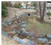
This innovative design allows a natural stream to function within a stormwater management facility and within close proximity to campus facilities.
